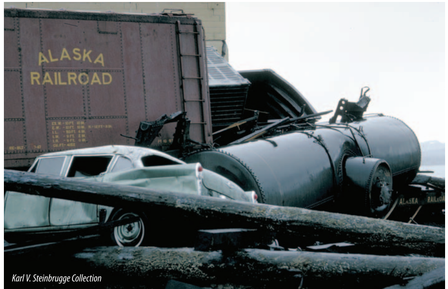
Damage in Seward following the 1964 earthquake. The waterfront area, railroad yard, and petroleum storage tank facilities were devastated by the tsunami.
