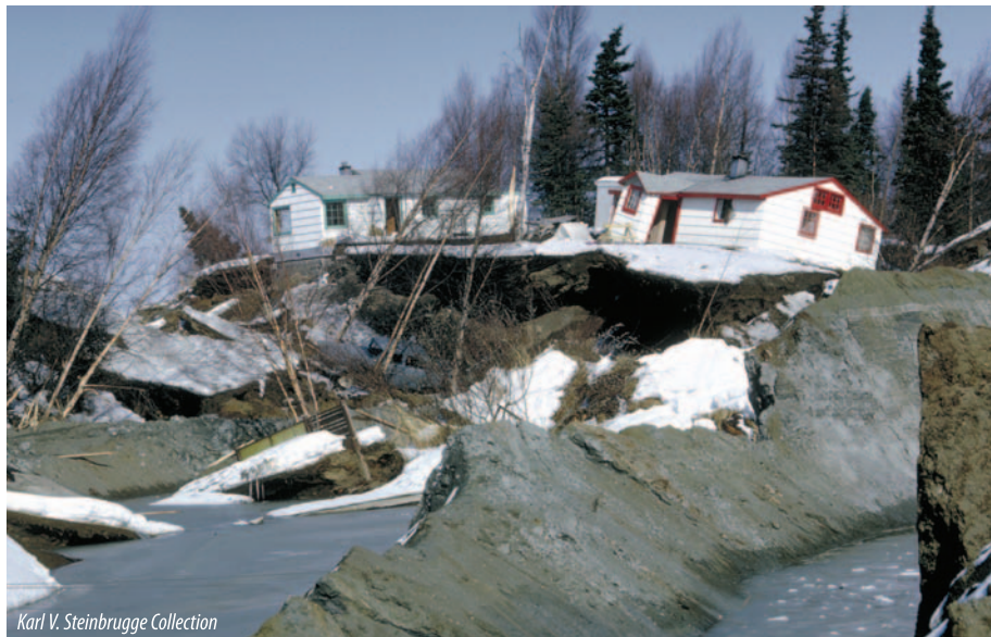
About 75 homes in the Turnagain Heights area of Anchorage were destroyed in 1964 by a massive landslide. This area is underlain by soil that flows like water when it is shaken.
