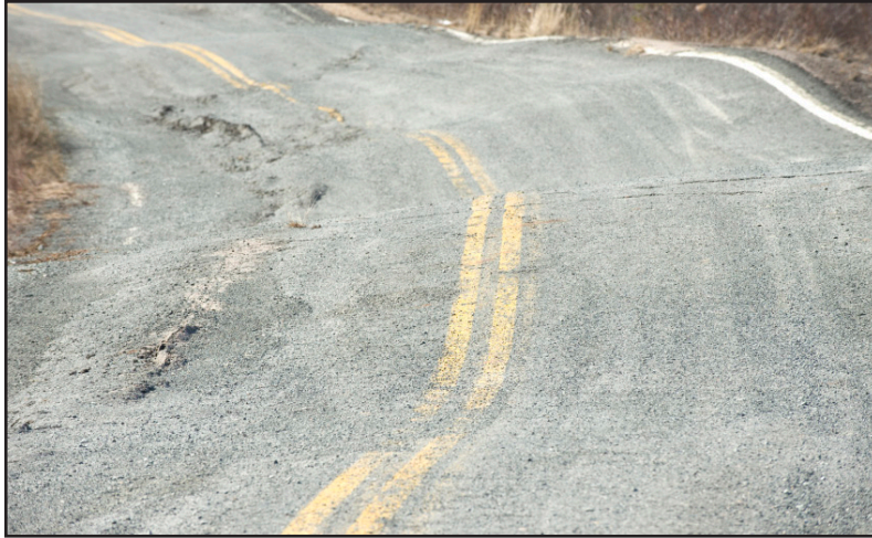
Permafrost thaw plays havoc with Interior Alaska roads. The road and its traffic put pressure on the ground below. Increased albedo caused by the dark road surface increases heat transfer. Photo from iStockphoto / RyersonClark.
