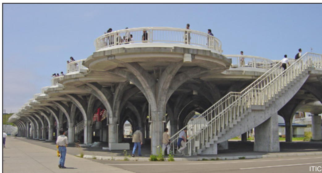
This elevated platform serves as a tsunami evacuation site on Okushiri Island in Japan. In tsunami-free times it also serves as a scenic view point.
