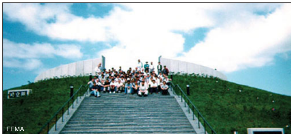
A berm is artificial high ground. This berm was built in Aonae on Okushiri Island in Japan.
